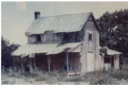
The Grove House (before Arnett's renovation)
