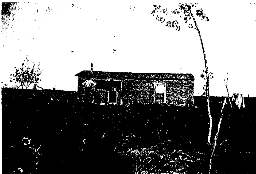
JESSE JONES SOD HOUSE BUILT ABOUT 1907 ON WEST SIDE OF SECTION 12-13-36 PICTURE TAKEN IN 1911
