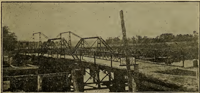
Iron Bridge, Reed's Ferry
